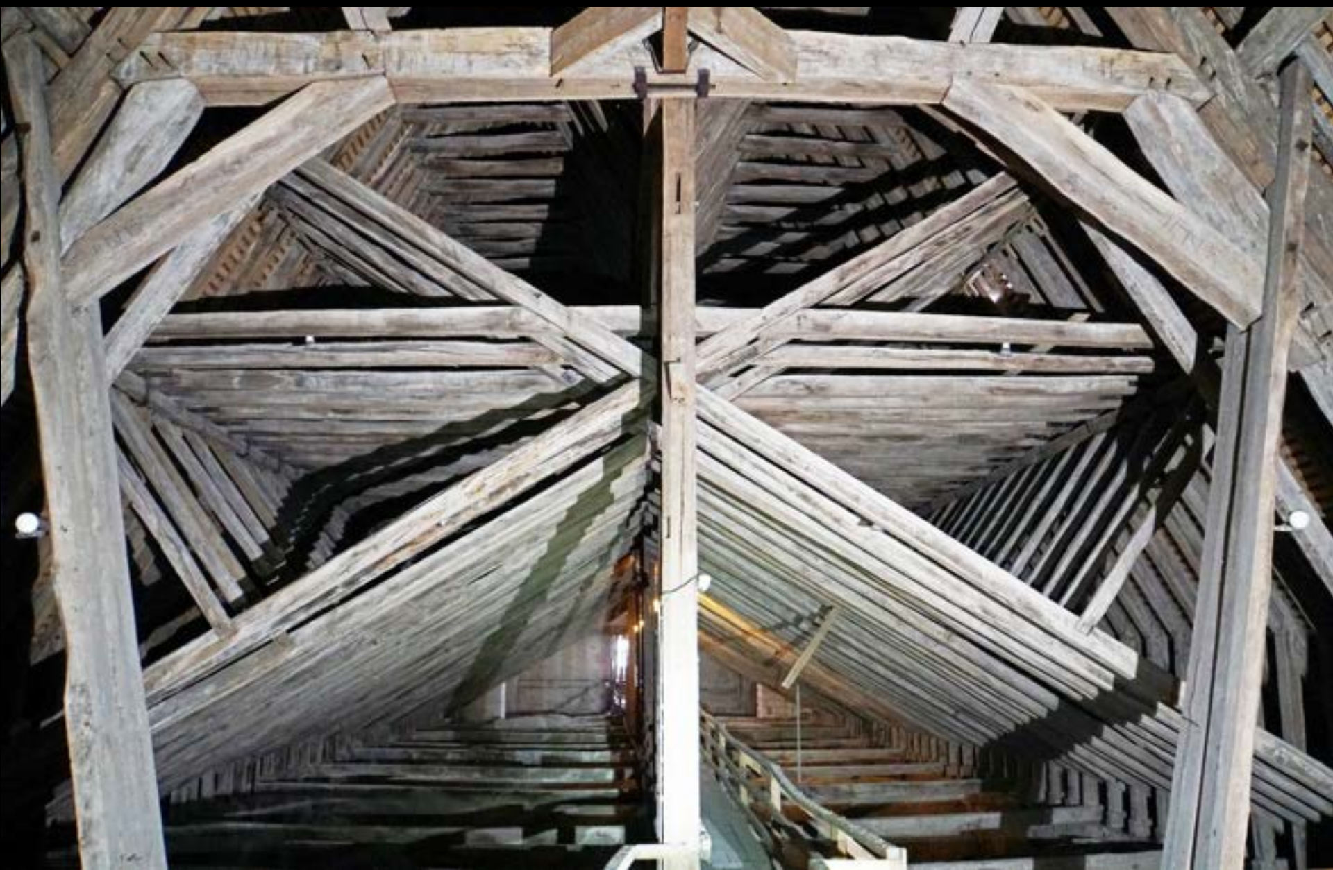
Sens, Kathedrale, Langhaus, Dach (1267d – 1293d)
